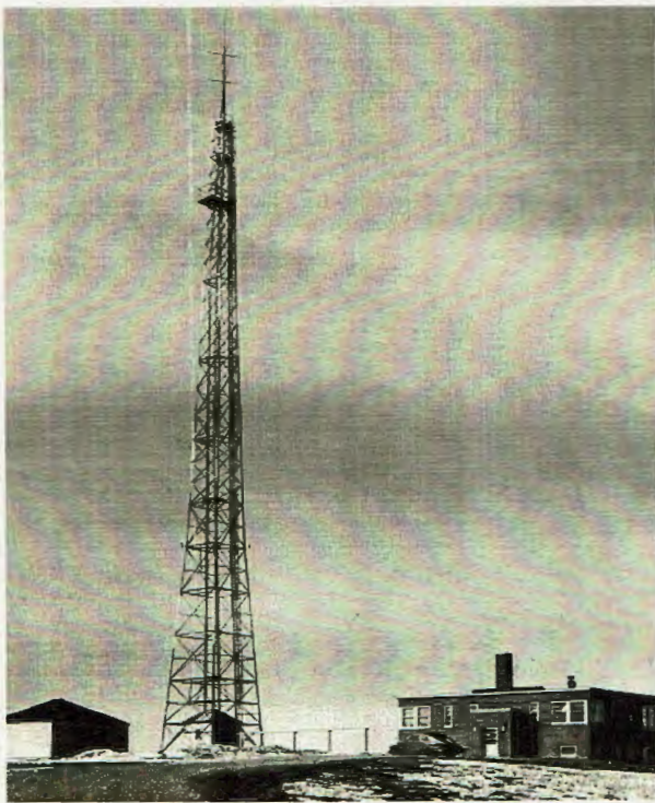
Journal Communication 200 ft. Tower South of Richfield Elementary School
