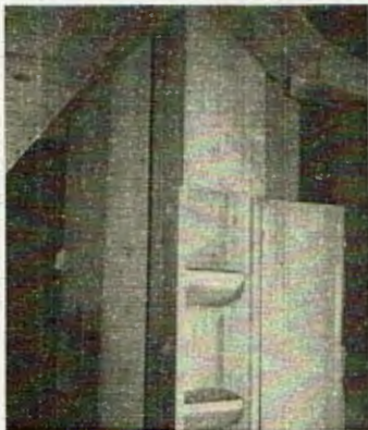
Oliver Evans Grain Elevators in the Messer Mayer Mill
